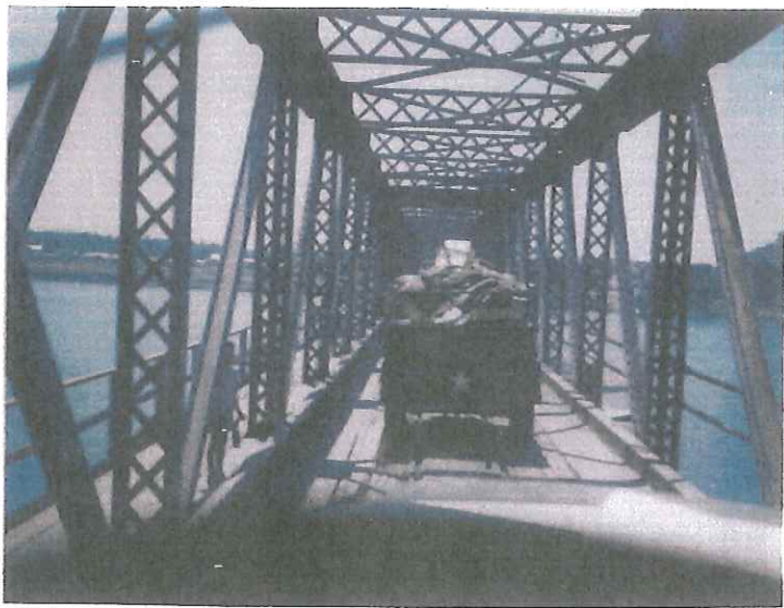
Hue, I believe this was a converted R.R. bridge
